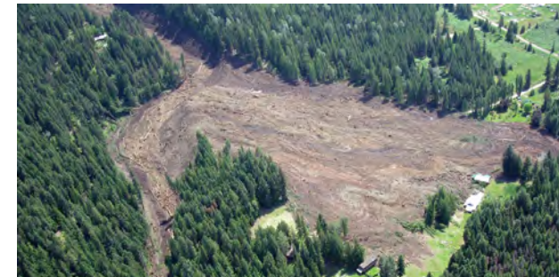
2012: A landslide severely impacted the community of Johnsons Landing, causing four deaths and completely destroying four homes.
